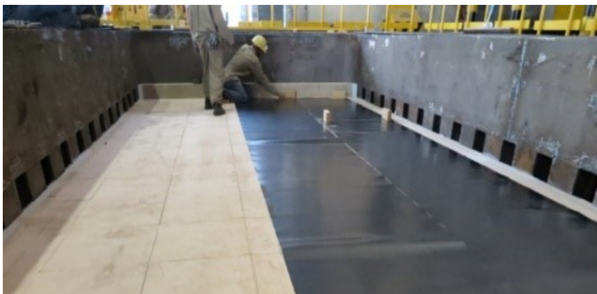
Figure 1. Cell construction using graphite foil.
